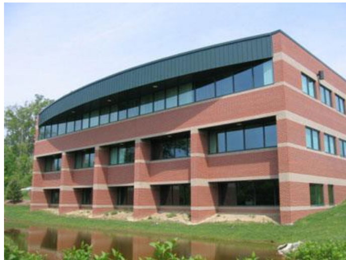
Figure 1: Stardock's Plymouth location. We bought this building in 2003ish
